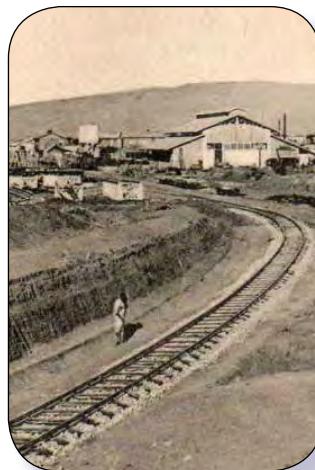
Railway in construction, Dirré-Dawa, Ethiopia. Photograph by Alfred Ilg, 1902.
